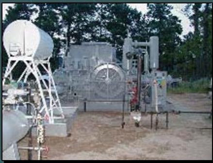
Gas compressors are used to gas lift water from wells. In this application compressors run 24 hours per day and for shorter periods. (<2 months)
