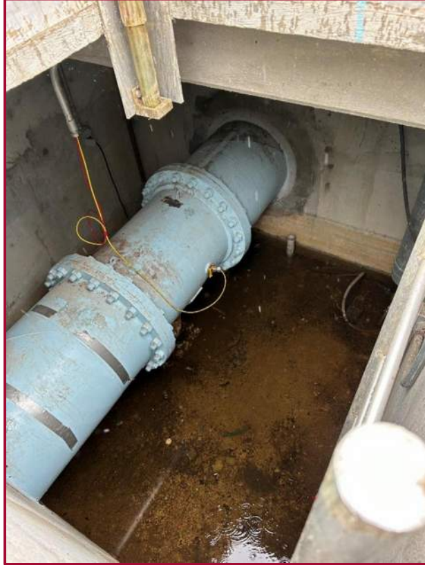
Photo 2.7 – Flow Meter Vault
