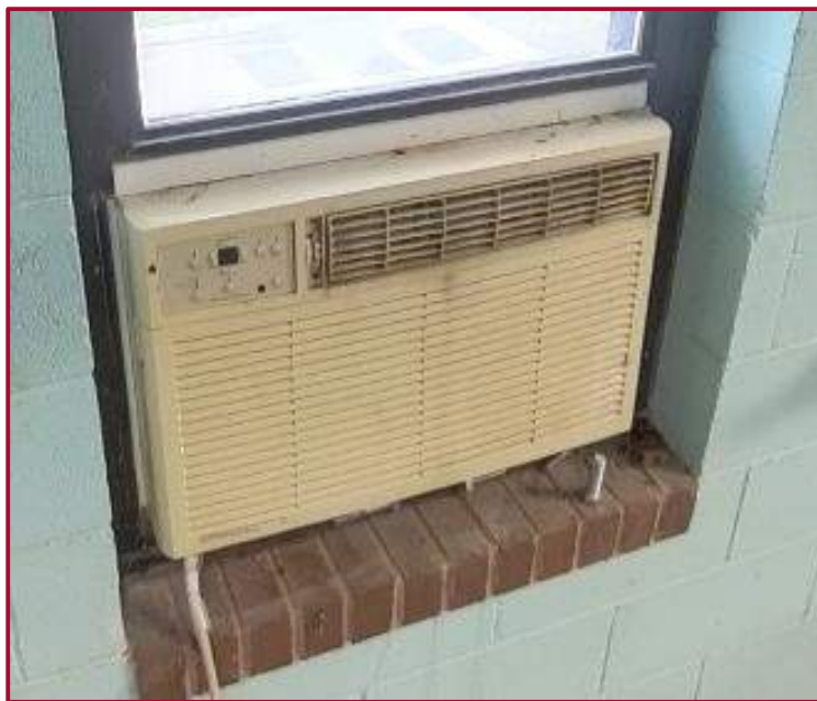
Photo 3.7 – Undersized A/C Unit
