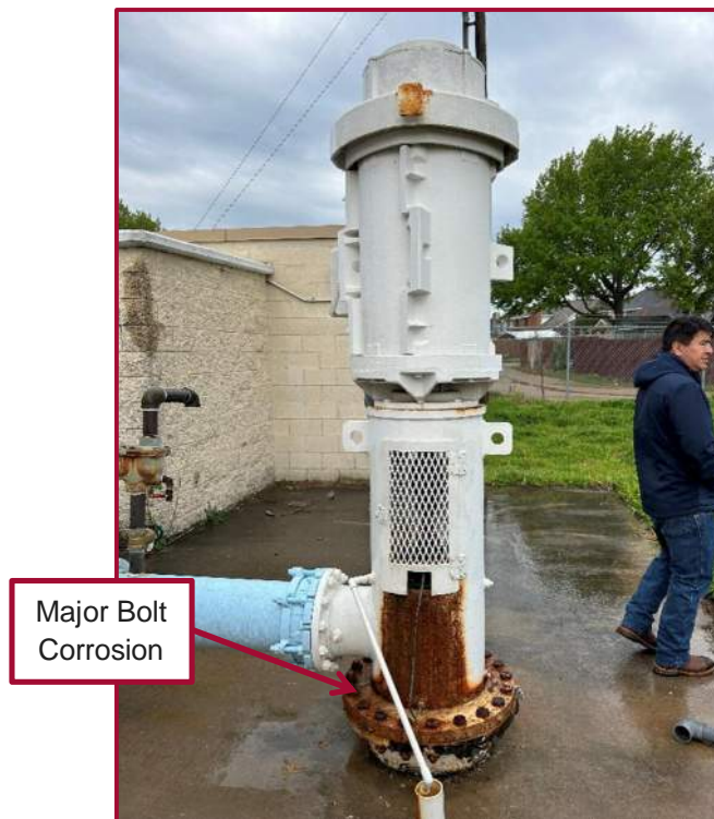
Photo 3.3 – Summit Pump Bolt Corrosion
