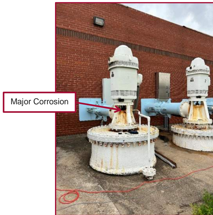
Photo 3.4 – Pump #3 Corrosion
