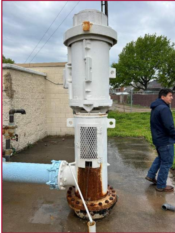
Photo 2.9 – Summit Vertical Turbine Pump
