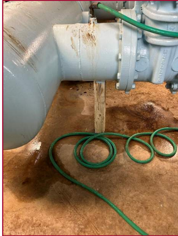
Photo 3.2 – Wooden Pipe Support
