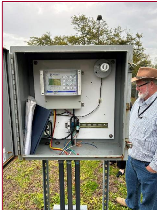
Photo 2.8 – Flow Meter Control Panel
