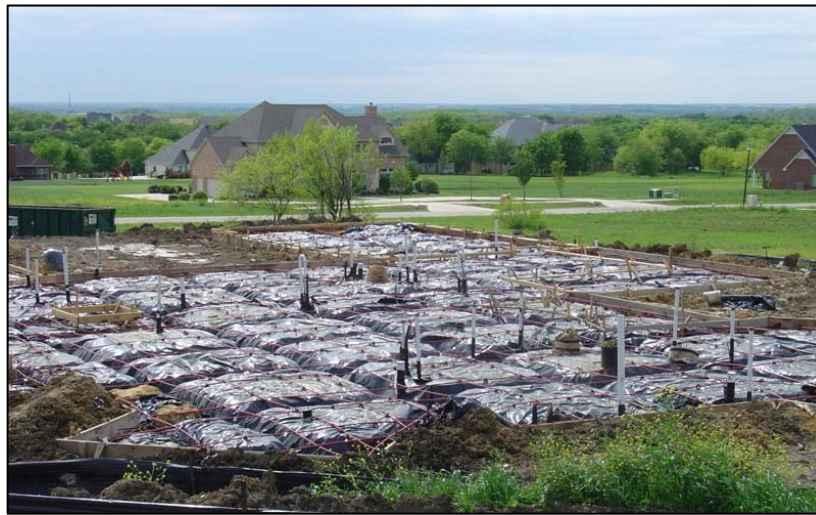
Foundation preparation on the Eagle Ford Shale
